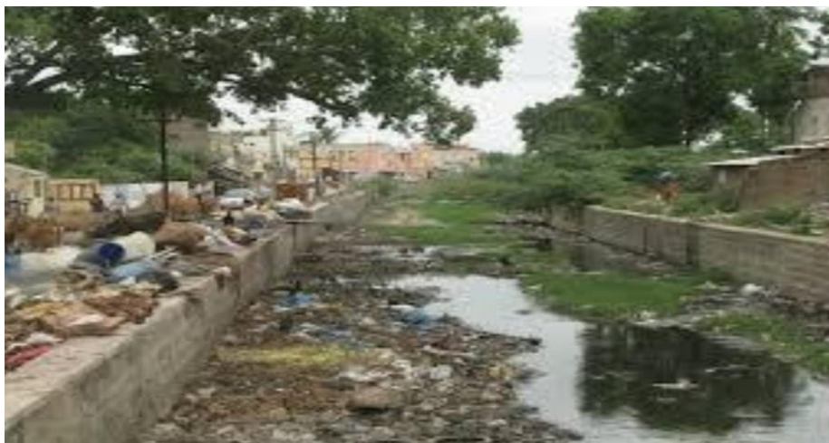
Fig.7: Main sewer of Kanker Khera (mohammadpur)
