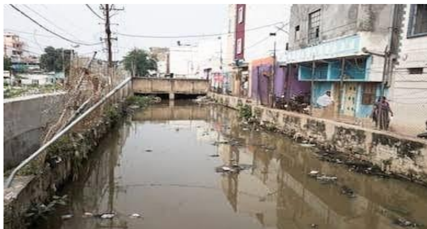
Fig.5: Municipal sewer of Begum Bridge
