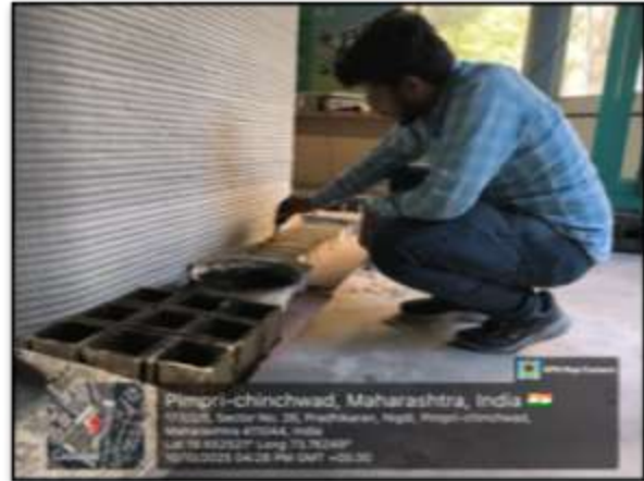
Fig. 4. Mixing of Concrete
