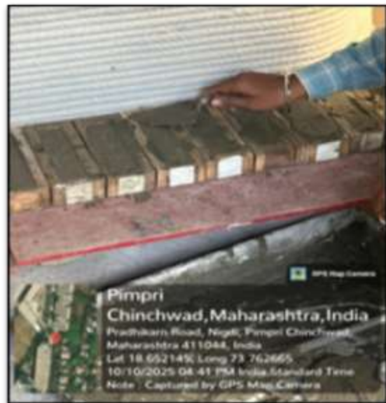
Fig. 7. Finishing is in progress
