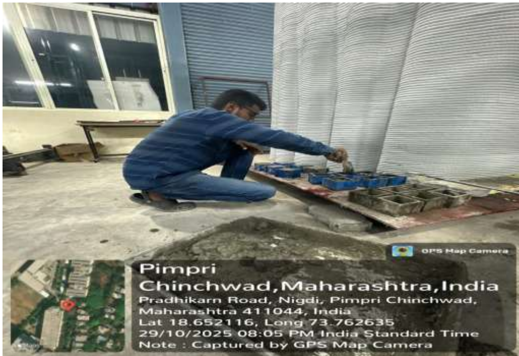
Fig. 3: Casting concrete into cube moulds
