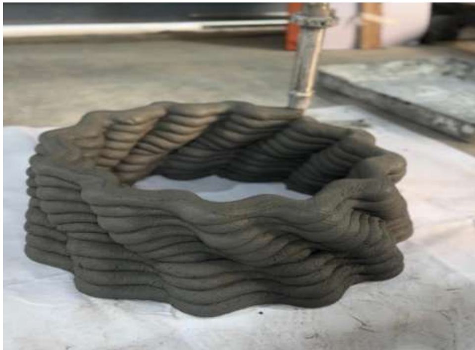
Fig. 17: 3D concrete printing process during trial
