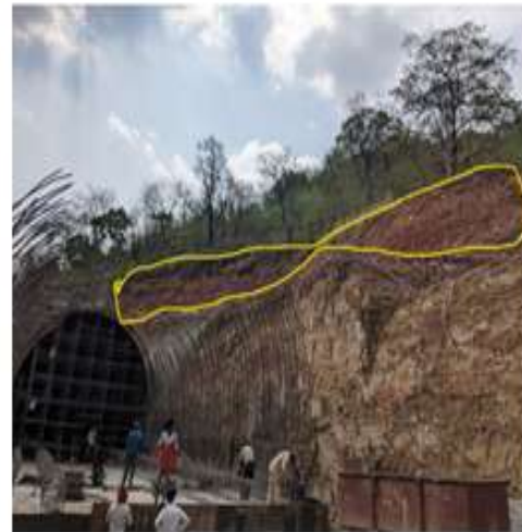
Figure 5: Unstable zone and Shale at Portal-2 of Tunnel No.2
