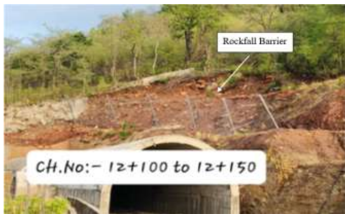
Figure 7: Installed Rockfall barrier at Tunnel Portal (Photo Source: RVNL Report)
