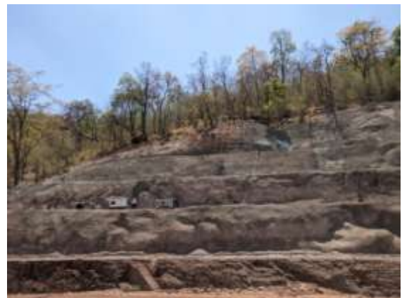
Figure 8: Cut Slope Stabilization
