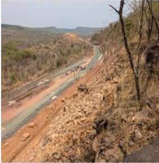
Figure 2: Slide from Ch.10+820 to Ch.10+960 Km with potential rockfall hazard.
