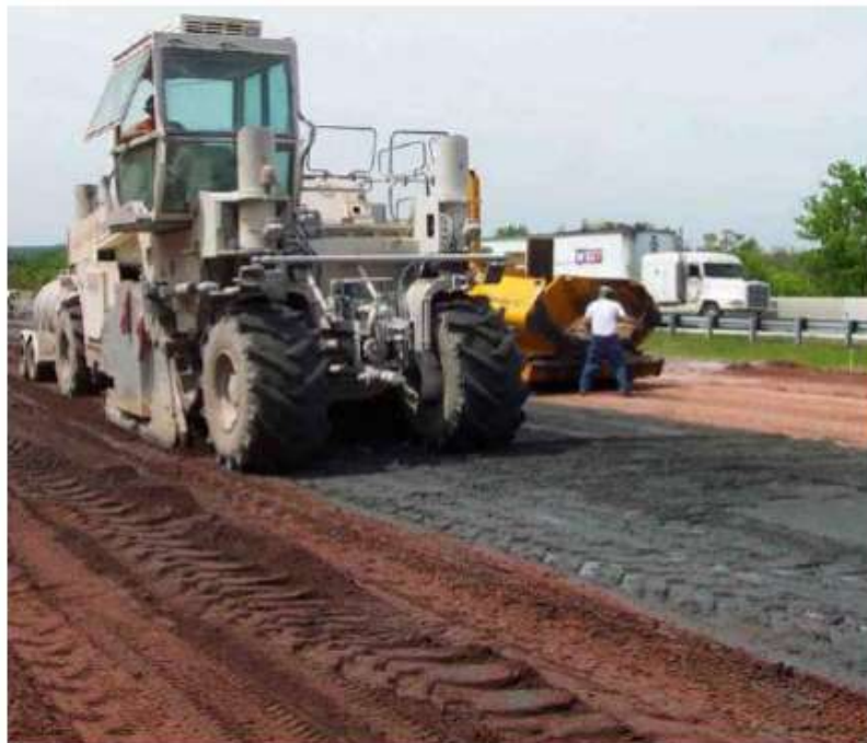
Figure 2: A road reclaimer mixes soil with moist conditioned fly ash. Soil to be stabilized shall have less moisture content; therefore, dewatering may be required. Soil-fly ash mixture cured below zero and then soaked in water are highly susceptible to slaking and strength loss. Sulfur contents can form expansive minerals in soil-fly ash mixture, which reduces the long term strength and durability.
