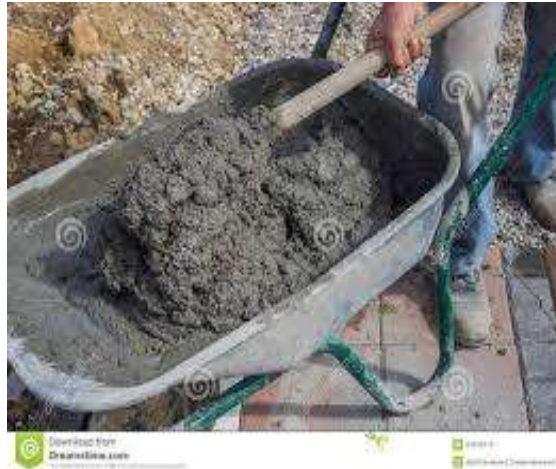
Figure 2 : Mixing of concrete
