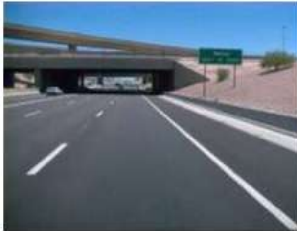
Figure 1: A sample bitumen material constructed road
