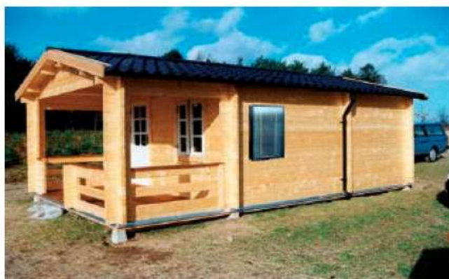
Fig.(6): installed on a cabin
