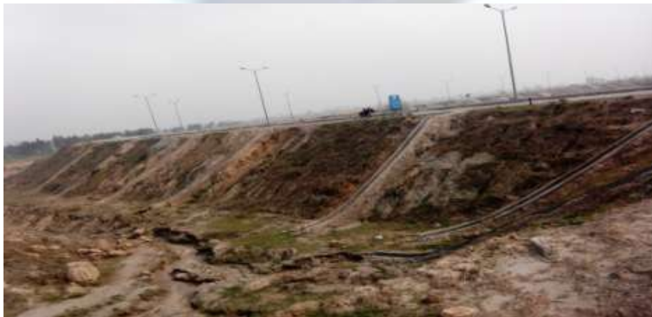
Figure - Slope with drainage chutes and vegetation
