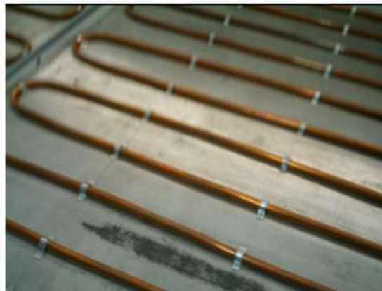
Figure 6. Aluminum sheet embedded with copper tube (CRCP)
