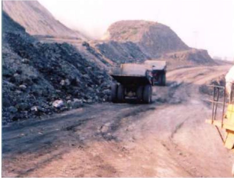
Figure 1: A typical permanent haul road
