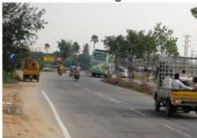
Fig 3: safety at night and adopting diversion as per IRC specifications
