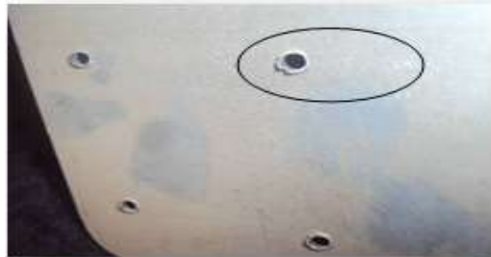
Fig- Not ok part (Hole Puncher /Crack)
